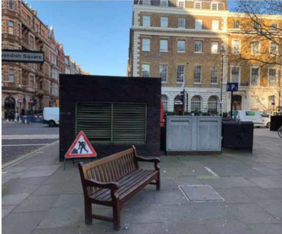
3M HIGH PLANT ENCLOSURE & STAIR- NORTH-EAST CORNER
