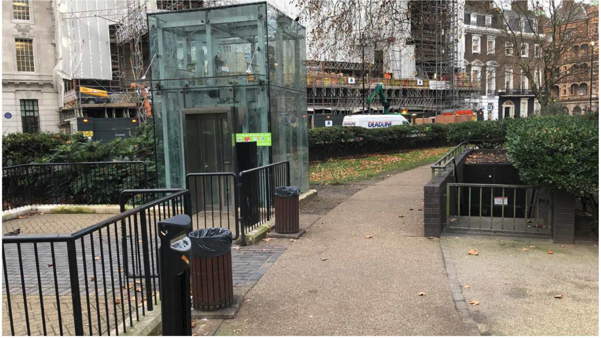
PUBLIC LIFT TO CAR PARK BELOW WITHIN GARDENS & ASSOCIATED CONTROLLED GATED ENCLOSURE & STAIR
