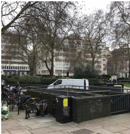
EXIT STAIR - NORTH WEST CORNER
