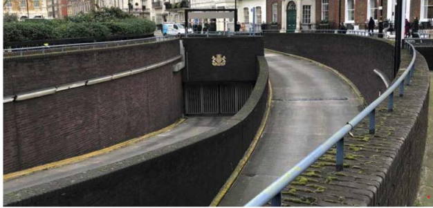
ENTRY & EXIT RAMPS TO S-E OF SQUARE WITH RAISED PARAPET WALL AND ASSOCIATED HIGH LEVEL ENTRANCE SIGNAGE & STAIR
